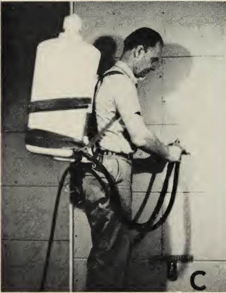
Fig. 28. Equipment used in "built-in pest control" at the time of construction of a building. A. electric blower for dusting attics via the attic "crawl hole"; B. dusting subcabinet voids; C. dusting wall voids; D. a fire extinguisher for blowing insecticide dust which may be used in place of the two other dusters shown in the figure.
